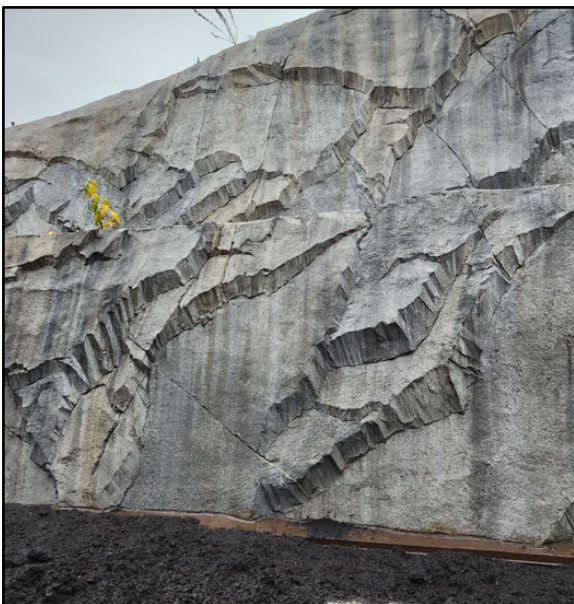
Drawing 3 – Picture of Rock Finish on Retaining Walls
